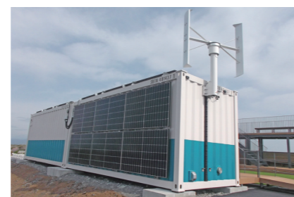
"N³ N-CUBE," which was adopted as independent power supply for the flood prevention center in Yoshida Town, Shizuoka Prefecture, Japan
