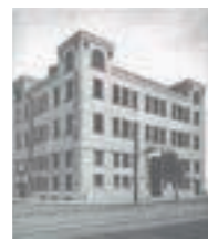
Old head office building
