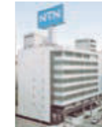
Current head office building
