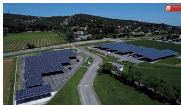
Solar panels installed in the Cevennes plant parking lot
